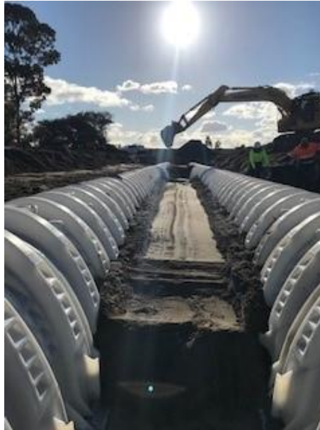
Pictures showing correct backfill method.
