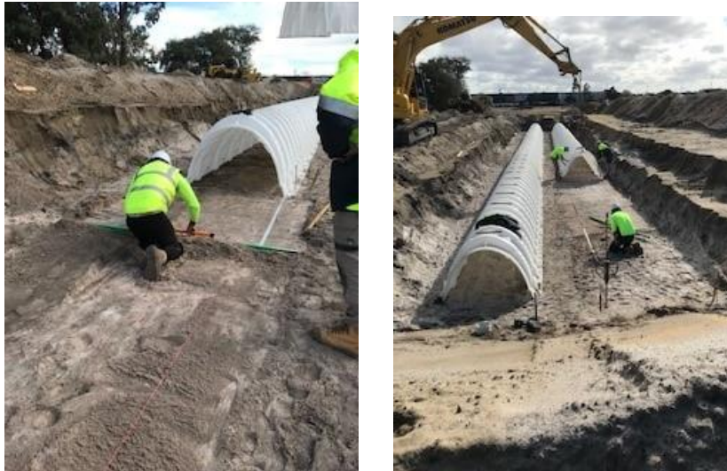
Pictures showing laying.
