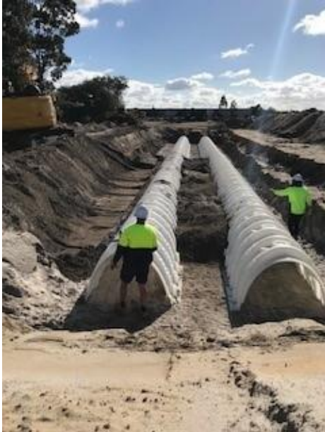
Pictures showing correct backfill method.
