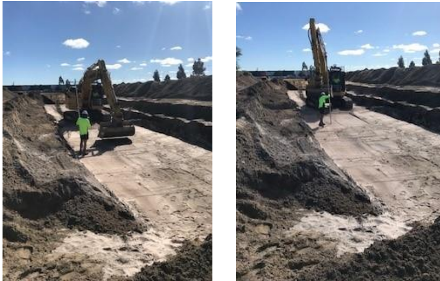
Pictures showing base layer compaction testing.
