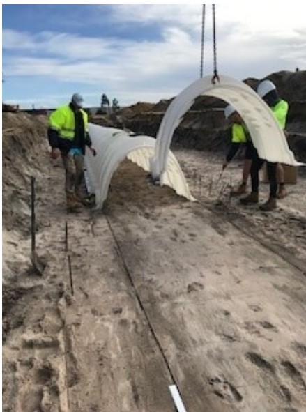
Picture showing laying.
