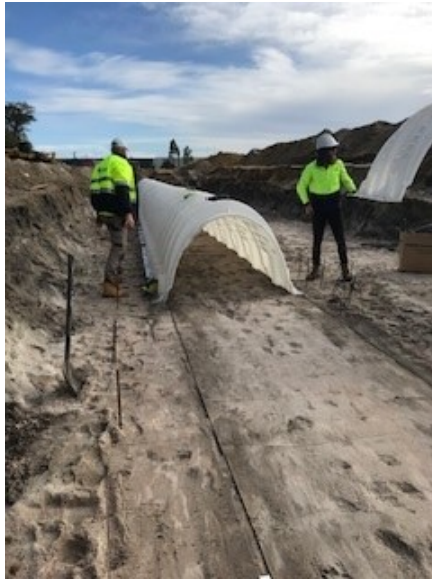
Picture showing laying.
