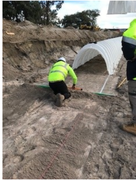
Picture showing laying.
