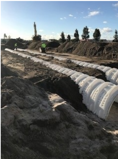
Picture showing backfilling.
