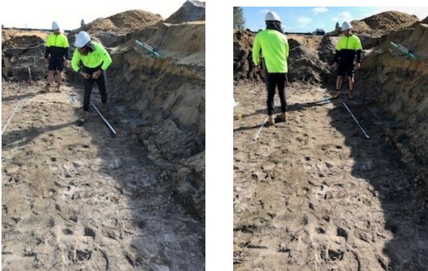
Pictures showing screeding.
